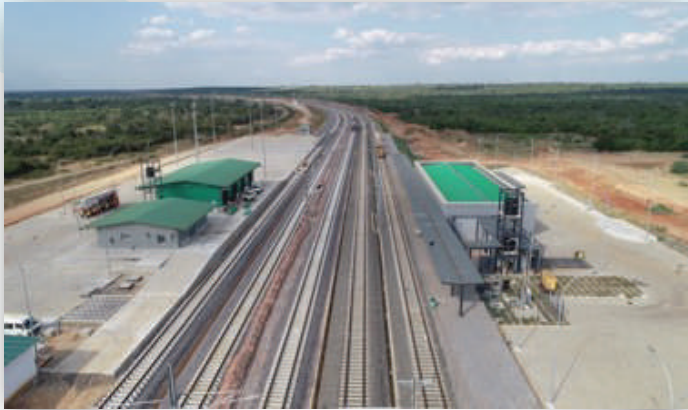
Standard Gauge Railway - Ruvu Station
